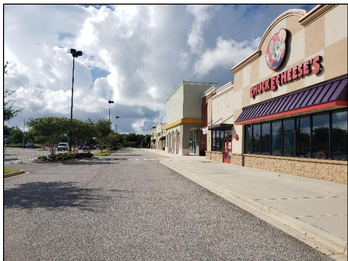
Figure 24. Former location of Resource 8DU15970, facing southeast.
