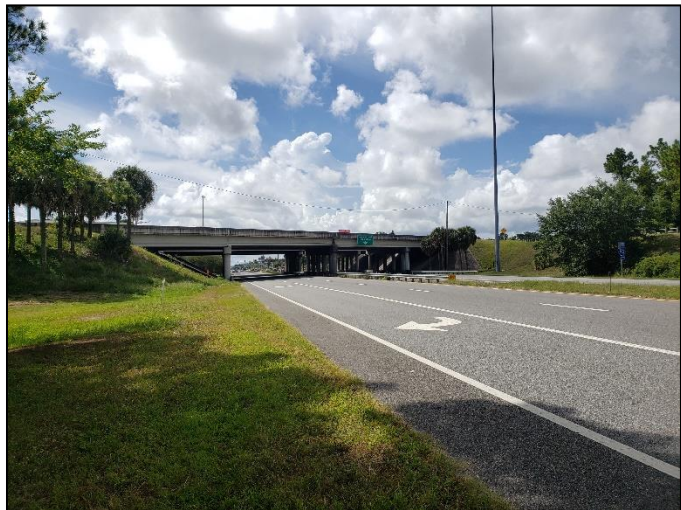
Figure 22. Resource 8DU18995, facing south.
