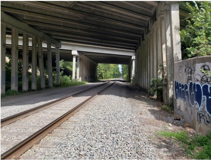
8DU17719_a Facing northwest
