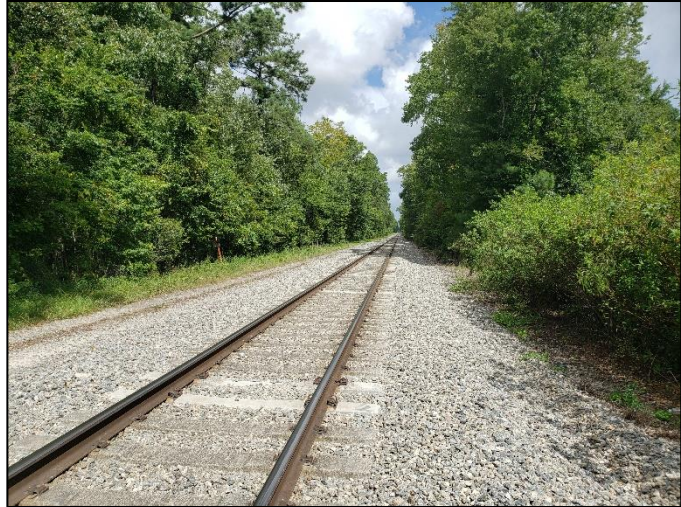
Figure 20. Resource 8DU17719, facing west.
