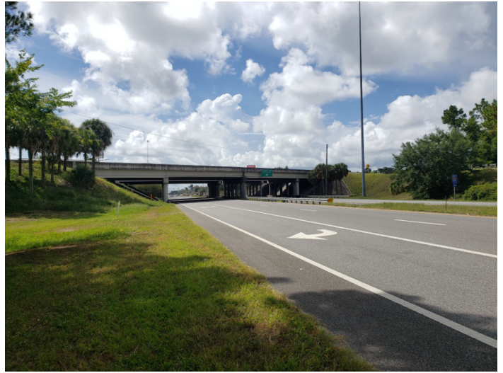
8DU18995_d Facing South
