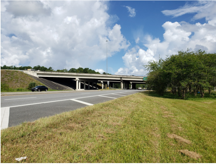
8DU18995_a Facing north
